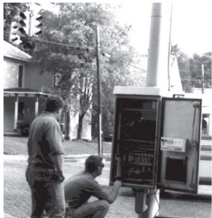
*Photo 2 Field testing of cabinet primary surge suppressor with a dark intersection. An extra person was needed to direct traffic during the time of no indications.*
